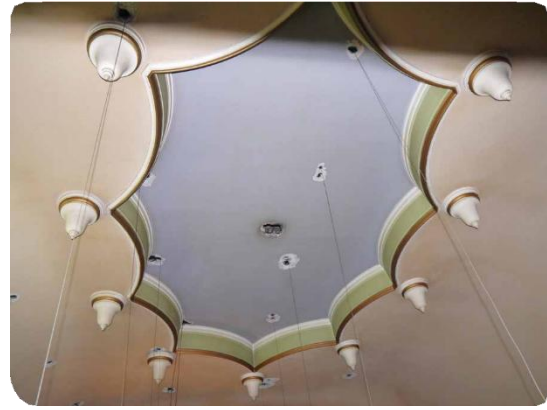
2019 view of the ceiling seen in the left hand image
