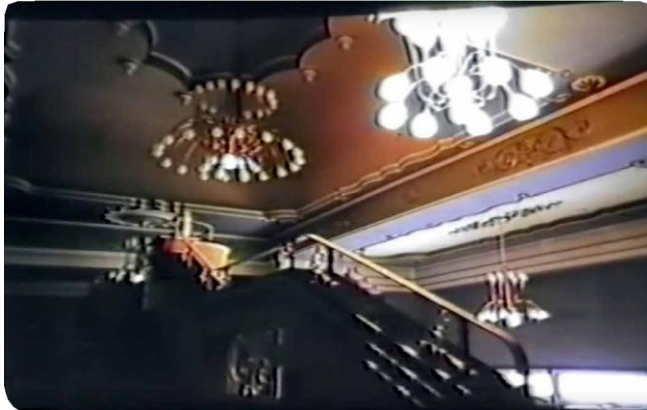
A view of the original entrance foyer ceiling
